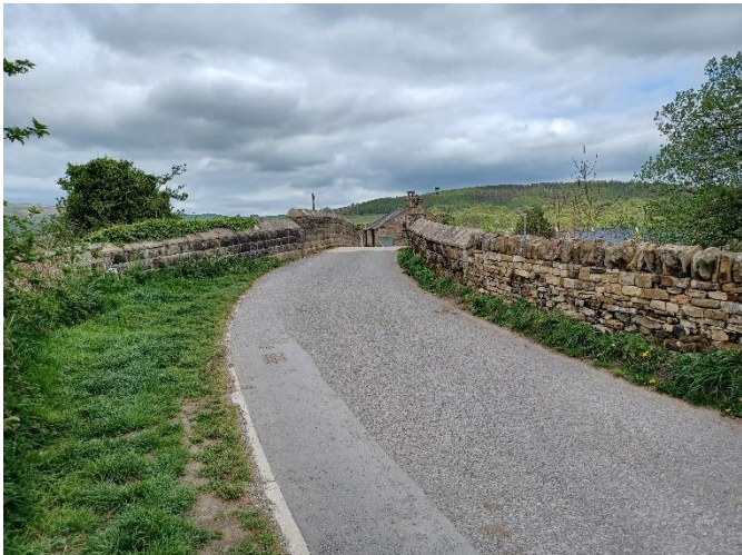
3. Bridge over the railway – Point B
